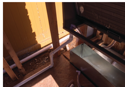
Figure 20: Condensate-tube installed
