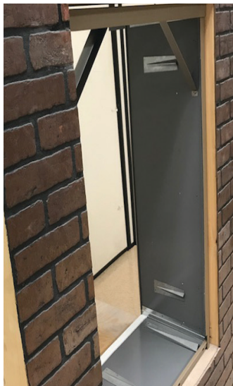
Figure 12: Fasteners attached through wall sleeve sides into the supporting wall
