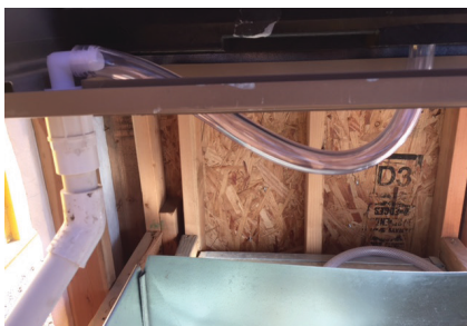
Figure 19: Condensate-tube installed
