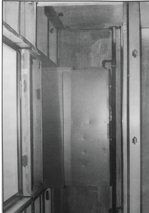
Figure: 27: Wall sleeve fastened to steel 2" x 4" studs with screws fasteners shot through sides of wall sleeve.
